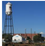
Alamosa Water Works
