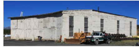
C&S Engine House
