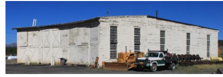
C&S Engine House
