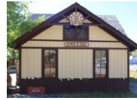
Creede Station End View
