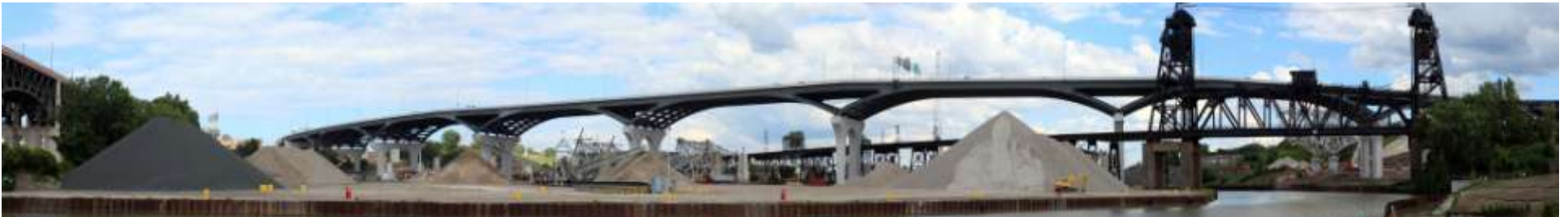
Voinovich Bridge - 6 Parts - 8h x 57w
