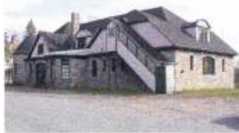
Stone Ex Station
