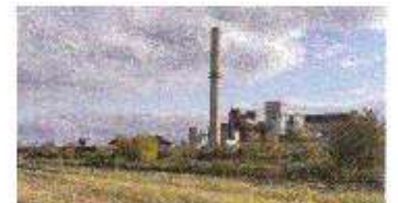
Stack Along the Track
