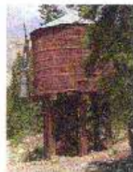
Tunnel Gulch Water Tank
