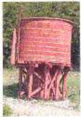
Boreas Water Tank
