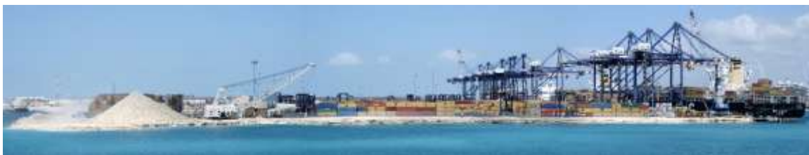
Done in Two Backdrops for Different Scales and Applications: Freeport Container Port Small – 44"W x 8"H – 4 Parts Freeport Container Port – 90"W x 14"H – 12 Parts
